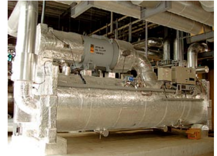
Inverter-type freezer at Fujitsu Hitachi Plasma Display that can be operated at high efficiency through control of rotational speed to match the seasons
