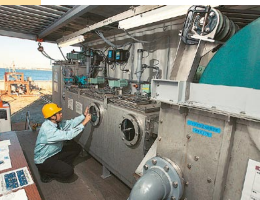
Test operation in Tokyo Bay
